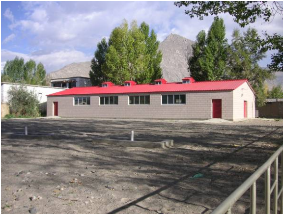
The animal house facility at TLRI
