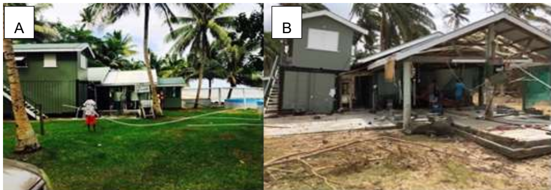
A= before cyclone Winston, B= after cyclone Winston
