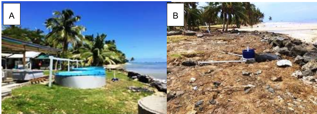
A= before cyclone Winston, B= after cyclone Winston
