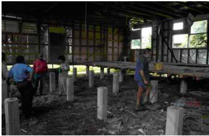
Figure 5. A ward at the hospital which had been destroyed by termites.
