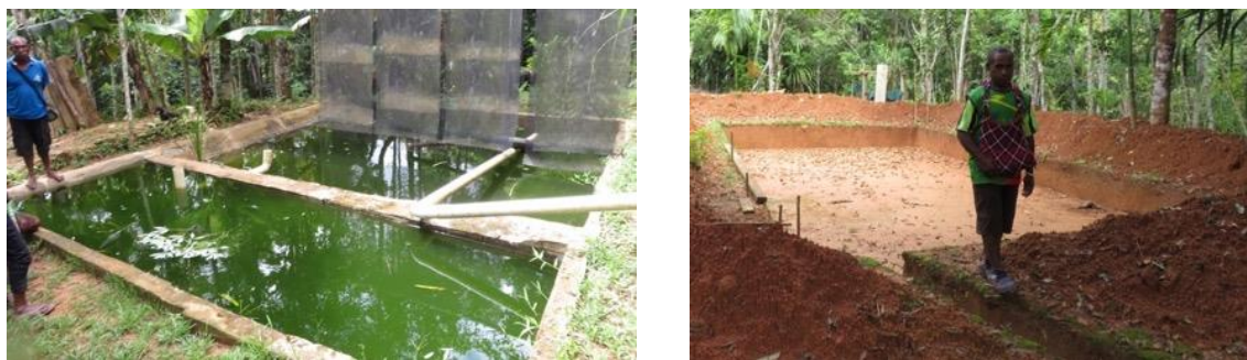
Figure 19. Completed (left) and under-construction tilapia ponds (right) in the Middle Fly.
