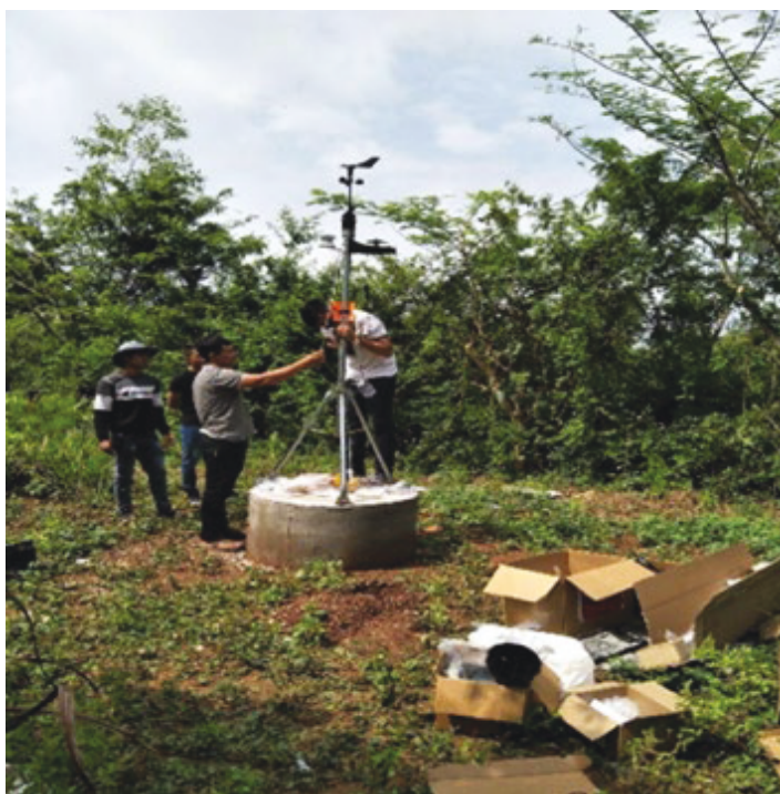
Figure 96. Weather station installation at National Meanchey University (NMCU)
