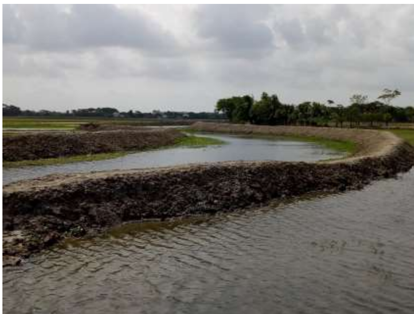
Figure 8.5 Re-excavated canal at Amtali. At the top corner there are rice field (Aus rice) grown using canal water.
