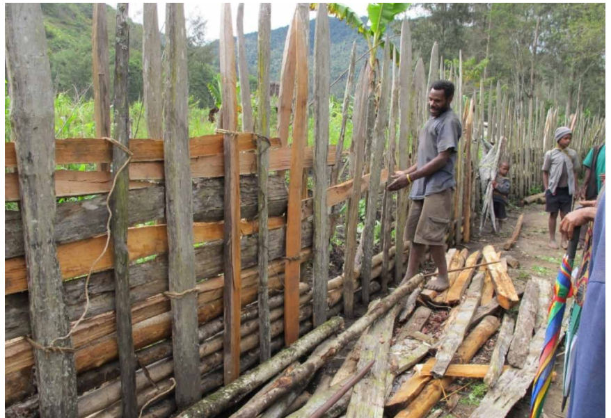
A timber fence under construction
