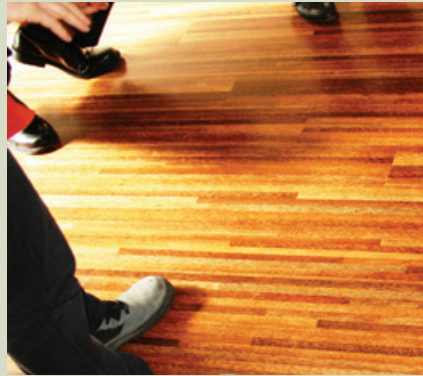
Figure 2.8. Engineered flooring combining sawn coconut and plywood.
