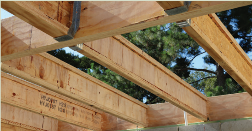
Figure 2.3. Structural beam products manufactured from rotary veneer.
