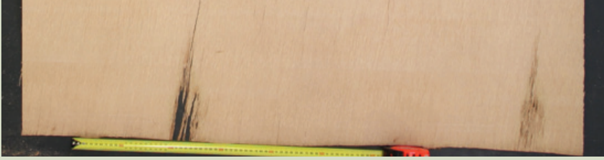
Figure 7.3. Fungal decay in cocoveneer.
