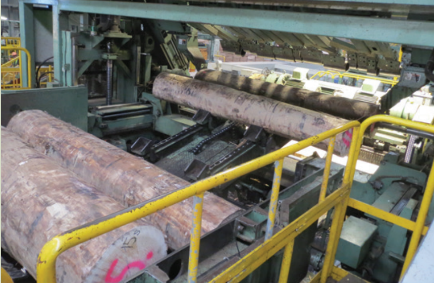
Figure 4.9. Log scanning ensures logs are positioned in the lathe spindles at the optimal location.
