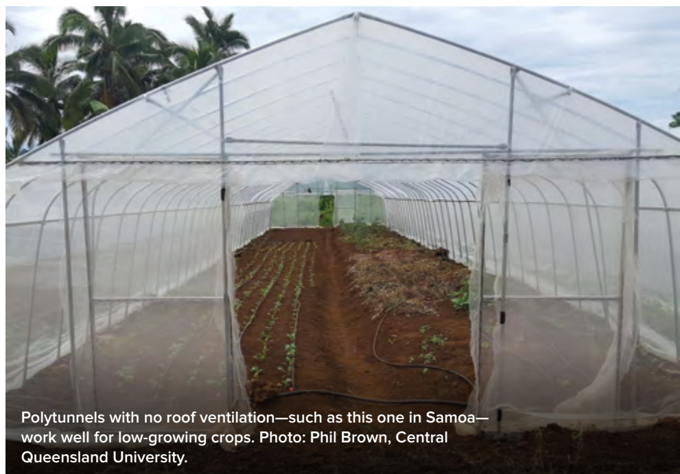
On the project demonstration site in Tavua, Fiji, a 360m 2 passively ventilated structure has been built. Photo: Phil Brown, Central Queensland University.
