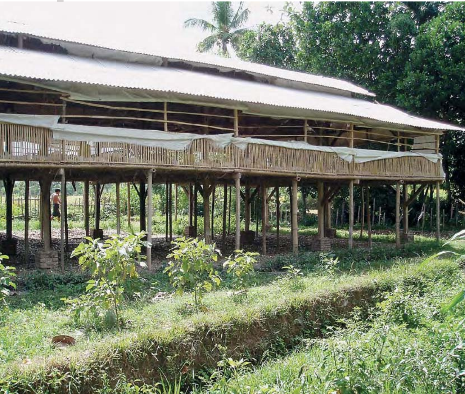
A family-run broiler farm outside Mataram, Lombok. In tropical climates, poultry sheds are elevated to allow ventilation.
