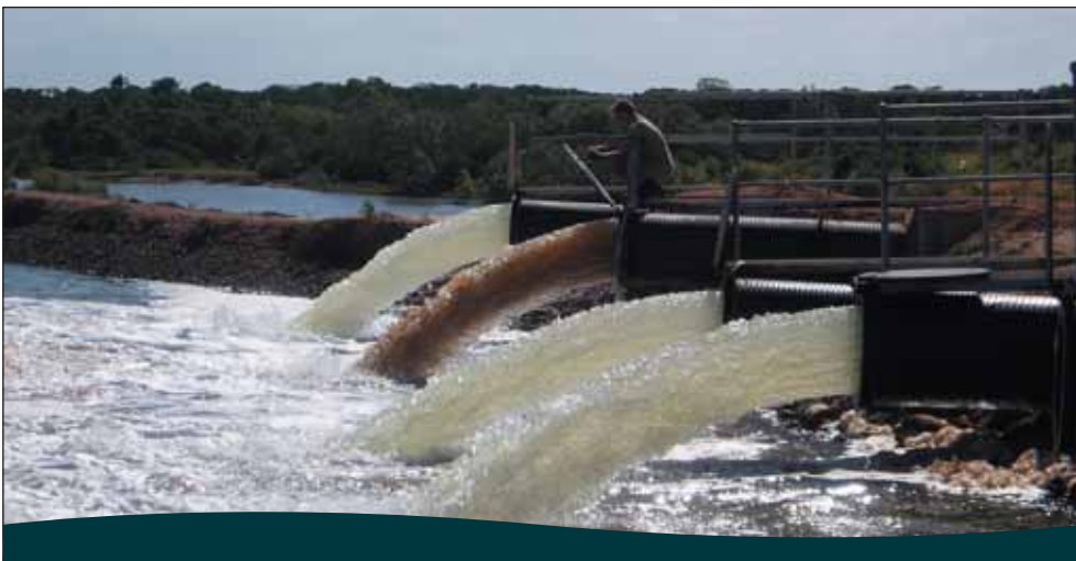
Figure 2.8 Pumping water into a reservoir
