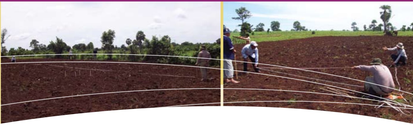
Figure 27. Squaring the site and lining up the pegs.
