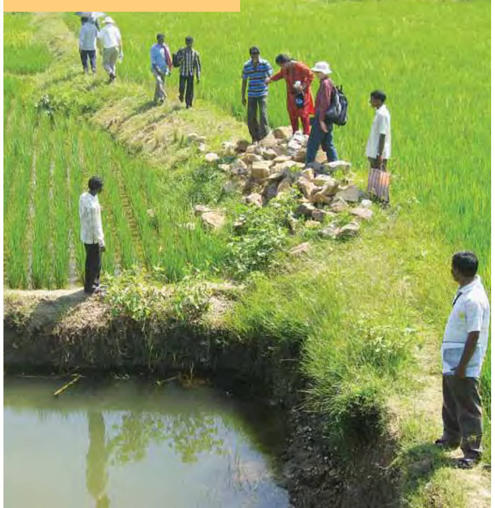
Farmers and project team inspecting a newly dug seepage pit in Pogro watershed.
