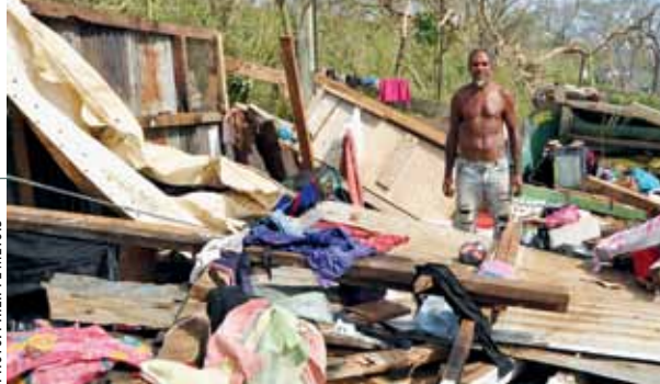
Aftermath of the cyclone in the Blacksands area, close to Port Vila.
