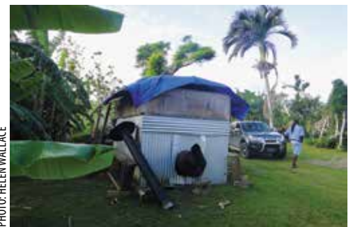
Damage to Vanuatu's industrial canarium-nut dryers and buildings in the wake of Cyclone Pam.
