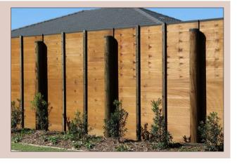
Figure 11.5. Preservative-treated plywood used for noise barrier construction.
