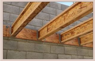
Figure 2.6. Structural beams combining rotary veneer flanges and oriented strand board web.
