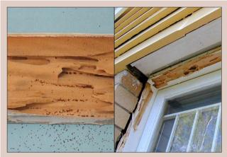
**Figure 11.1.** Termite damage to wood.
