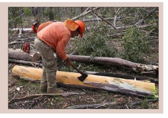
**Figure 3.18.** Removing bark with the cutting face of the axe.
