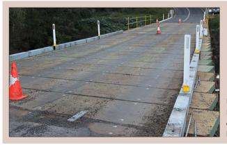
Figure 2.11. Bridge deck—an example of a veneerbased mass panel.
