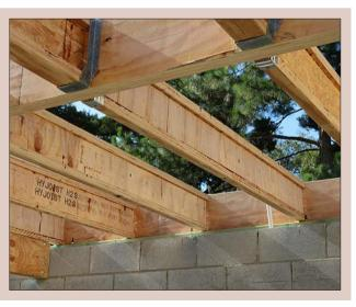
Figure 2.3. Structural beam products manufactured from rotary veneer.
