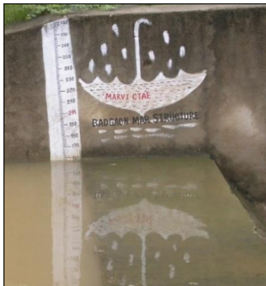
Figure 4. The Badgaon check dam water level measuring gauge with water level exceeding check dam crest level.
